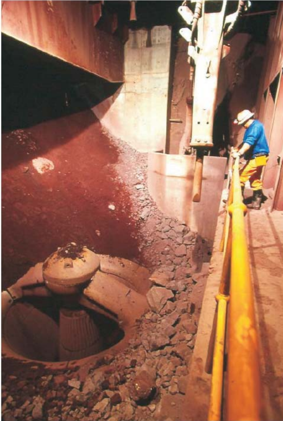
FIG 3 - Rail dump station ROM pocket and gyrotory crusher.
