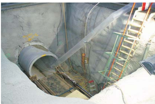
Somerton Road Pipe Jacking
